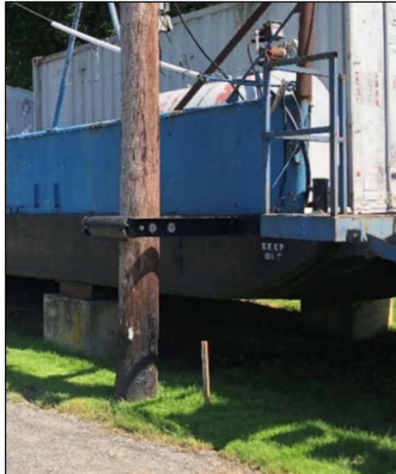
Figure 4-13: Floats Rail to Accommodate River Water Fluctuation
