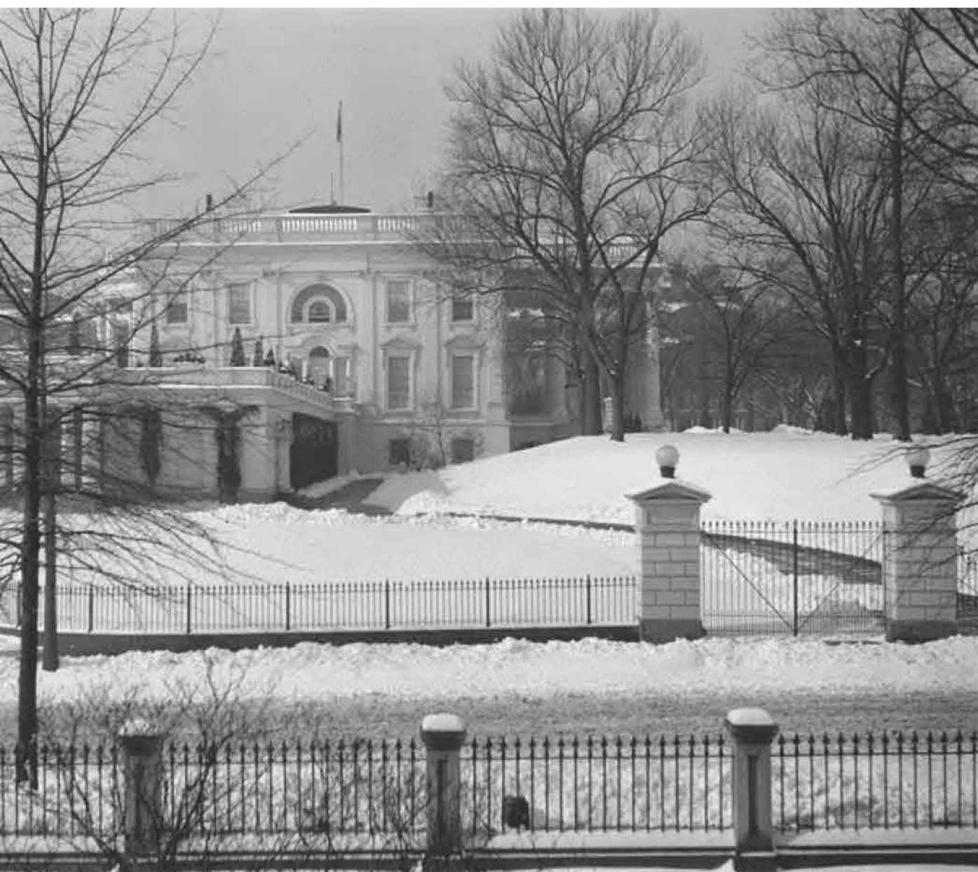
Photo ca. 1900 East Executive Avenue - iron fence & gates
