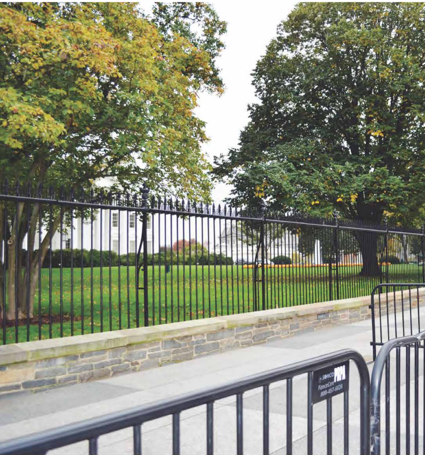
North side along Pennsylvania Avenue Existing
